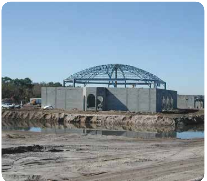
St. Timothy Church while under construction.
